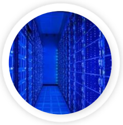
Microgrids, Data Centers, Emergency Power, & Fast-Start Capable
