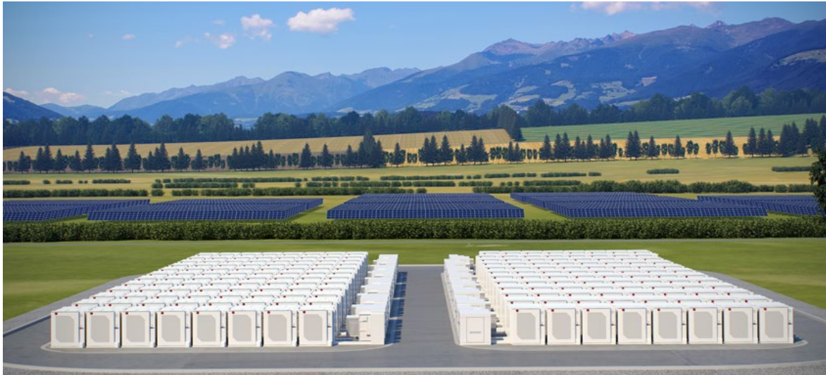
Storage system centralized adjacent to PV field
