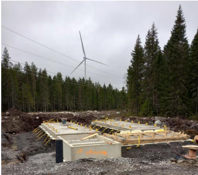
April 2023 Building the foundation
