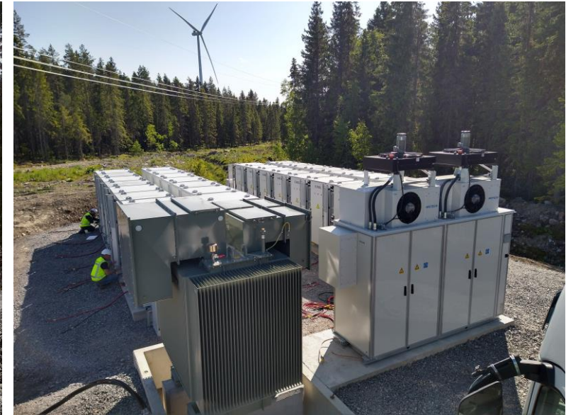
June 2023 Installation and cold commissioning
