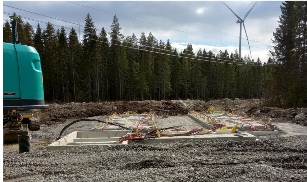
May 2023 Cabling works on going
